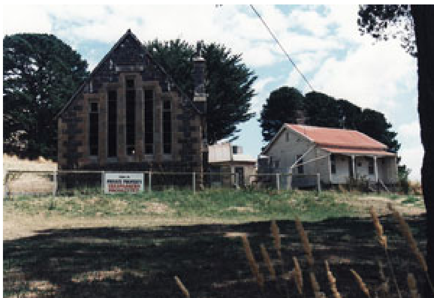
Former Weatherboard School & Residence
