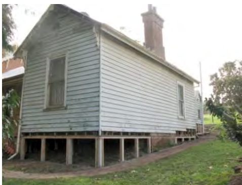
Above - After the re-stumping had finished.
